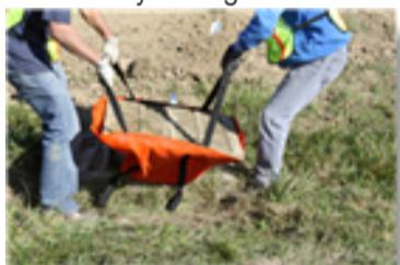
The Dandy Sack is made in the USA and features internal straps that cradle the grate for added support and security when installing and removing for maintenance. It comes in three sizes, it doesn't need rebar and its long-wearing design makes it one of the most cost effective sediment control solutions on the market today. [Click here](#) to see it in action!
